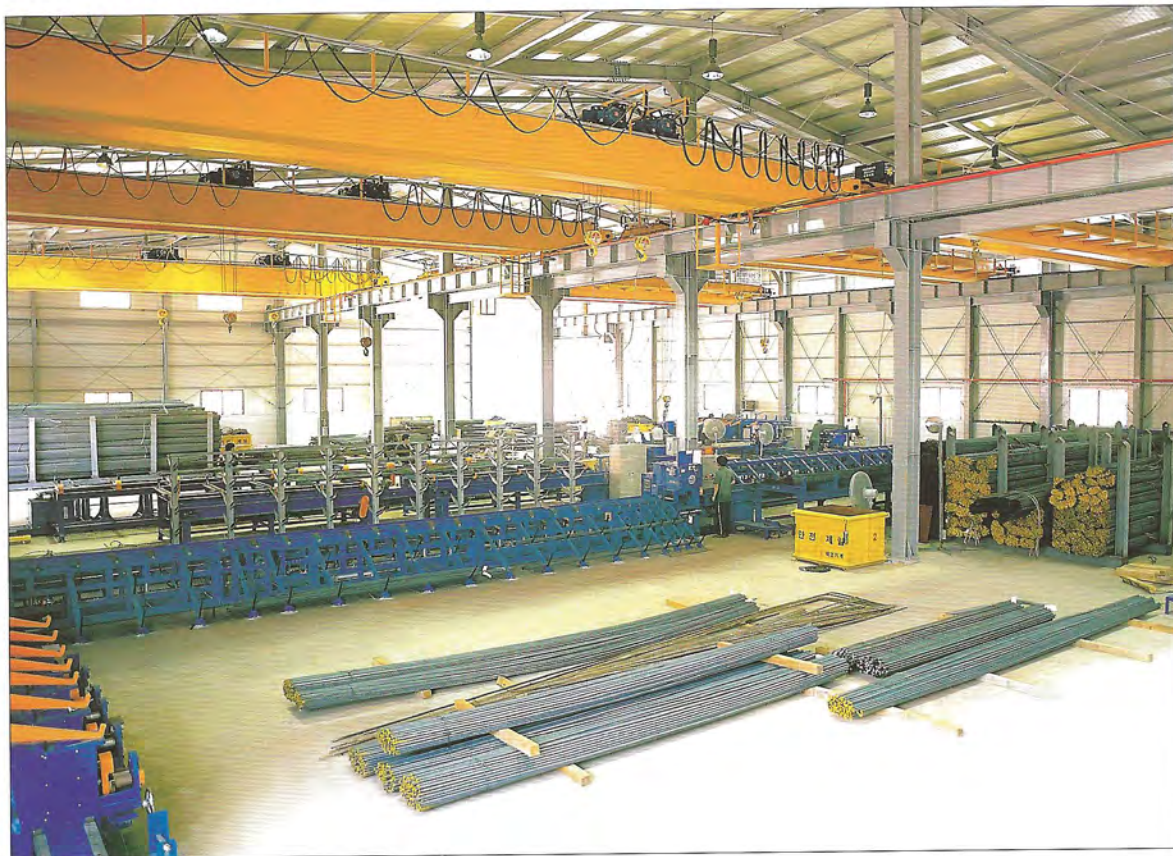
3rd Rebar Processing Factory - Inside view
