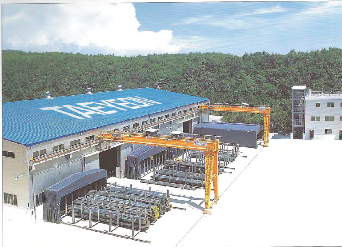
2nd Rebar Processing Factory
